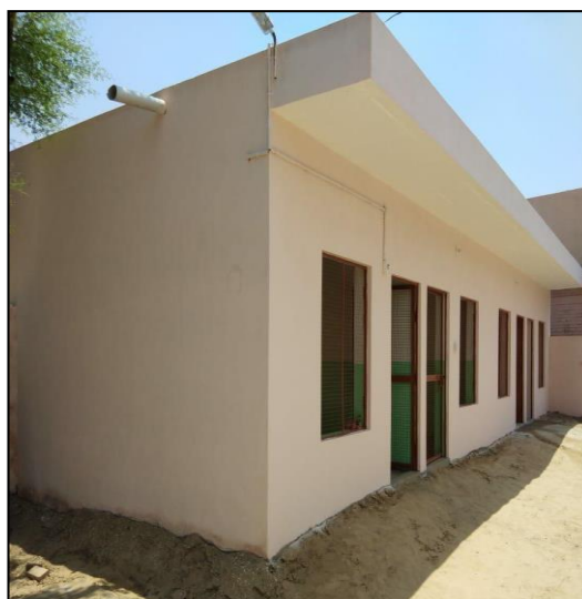
Figure 6.2 :- Rescue Center in Range complex, Abohar:
