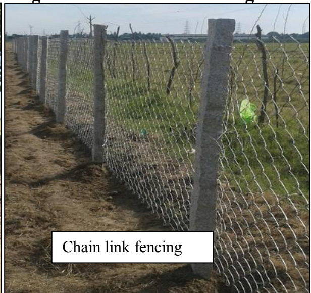
Figure 5.9 Chain link Fencing
